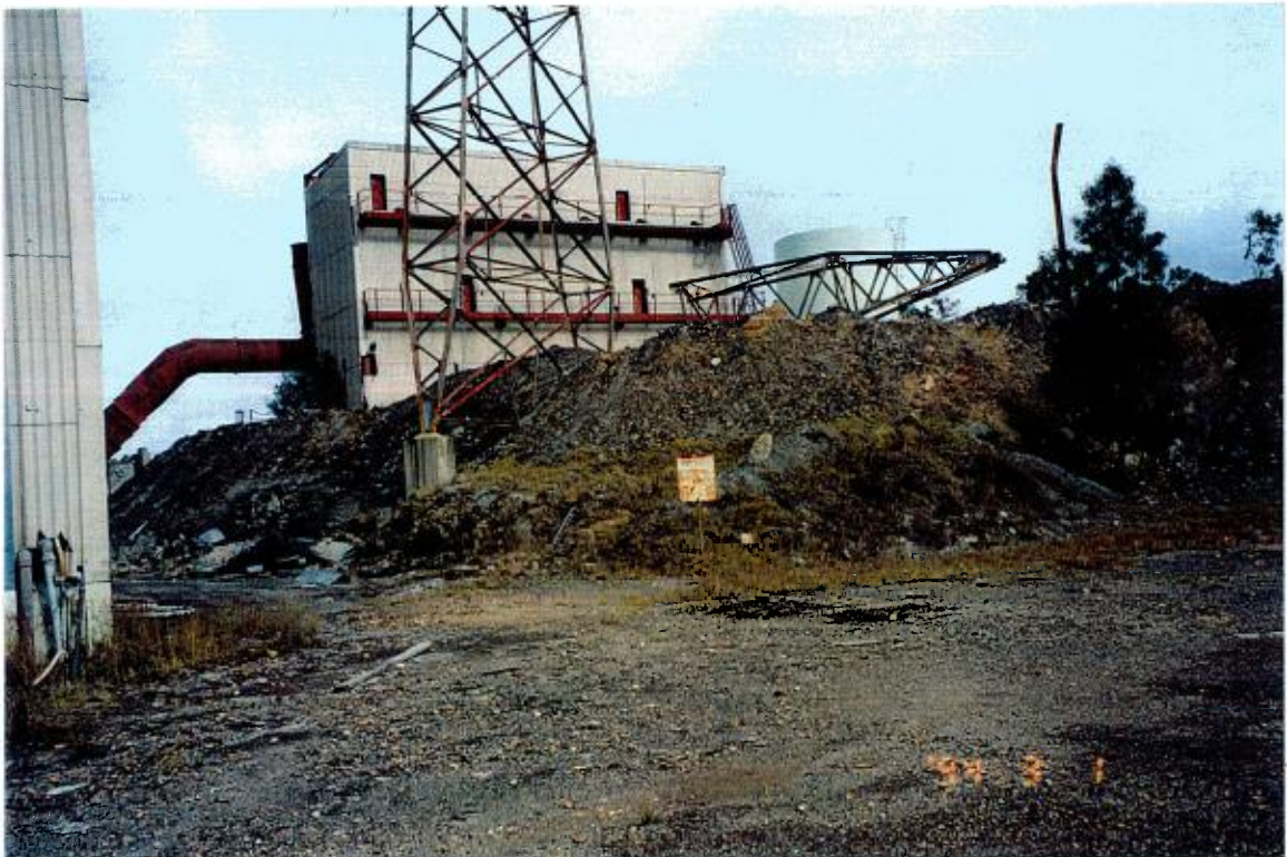
Drying House, of three levels, containing filter bags and highly contaminated.
