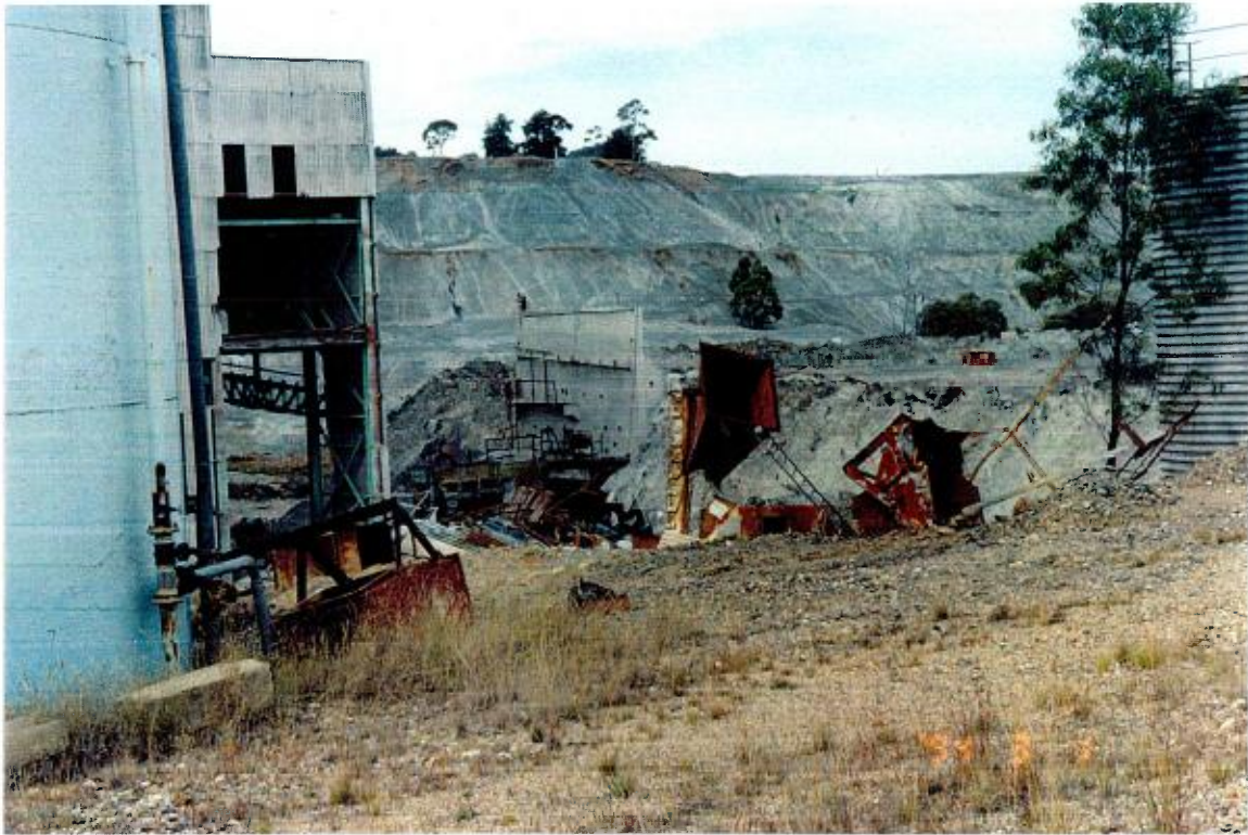
View from the west of the remains of the Crushing Plant.
